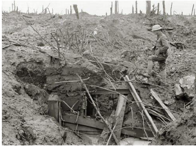
Leslie Blake inspecting the effect of a 9.2-inch British shell on a German reinforced concrete dugout on Hill 60 (Ypres), Menin Road Area. Photograph by an unknown photographer and dated August 1917. © Australian War Museum.
